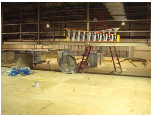
Dance Floor Scaffolding - Theater
