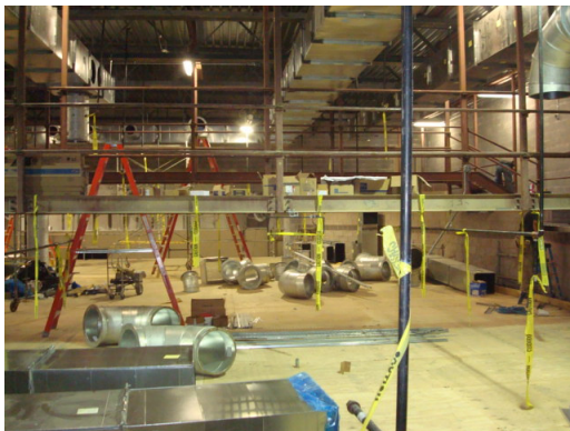
Auditorium Scaffolding OH Work
