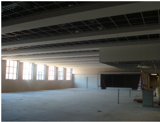
Media Center – Ceiling Soffits
