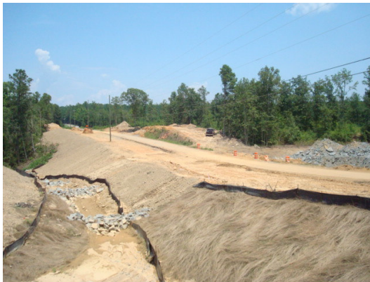
Bone Dry Road – Backfill of Installed Storm Lines
