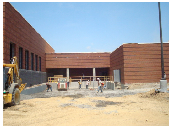
Loading Dock Concrete Prep
