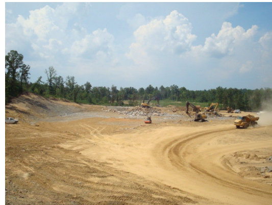
Rock Removal along Northwest Corner of Site (Future Baseball Field)
