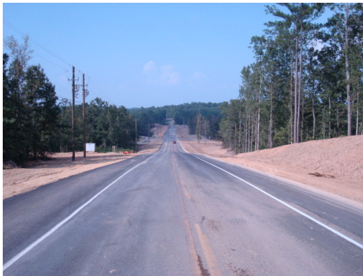
Bone Dry Road – Asphalt Base on East & West Shoulder
