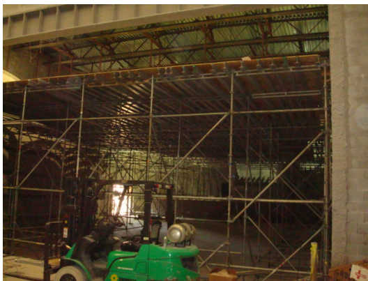
Dance Floor Scaffolding Installation - Theater
