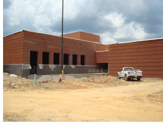
East Side of Area B / Loading Dock
