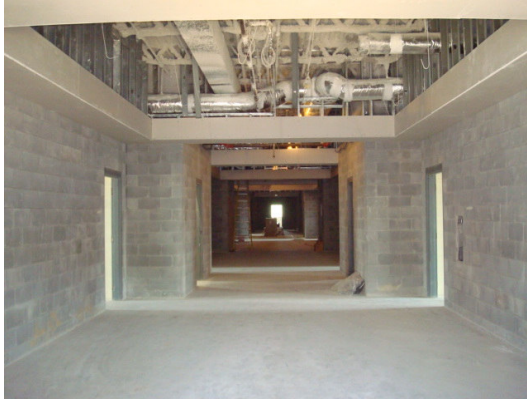
Area "F" Lvl 2 – MEP Overhead & Ceiling Framing
