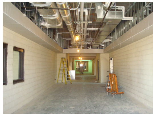
Area "E" Lvl 1 – MEP Overhead, Ceiling Framing, & Block Fill
