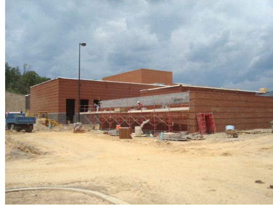
East Side of Area B / Loading Dock
