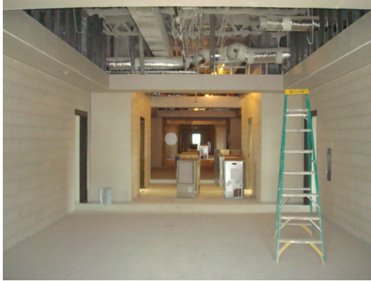
Area "F" Lvl 2 – MEP Overhead & Ceiling Framing
