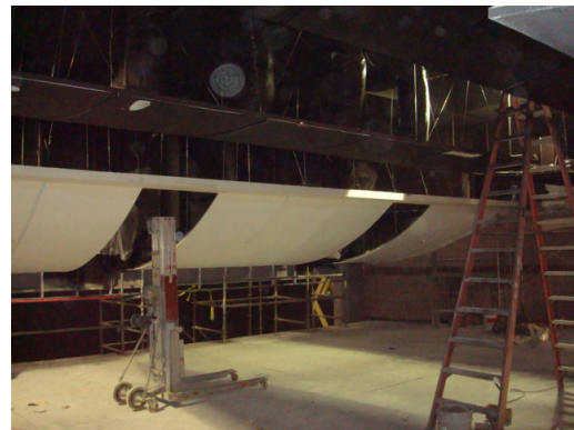
Radius Cloud Framing at Auditorium with paint
