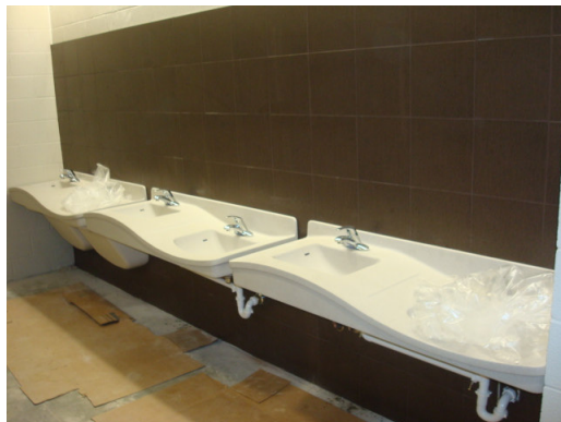
Bathroom with wall tile and sinks installed.
