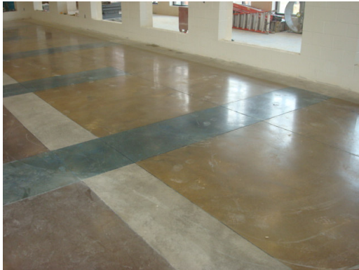
Cafeteria polished concrete.
