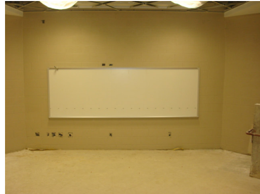
Markerboard installed in Lecture Hall.
